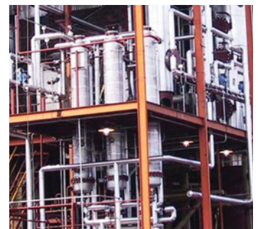
Cooled product is sent to carbon adsorbers to reduce color
